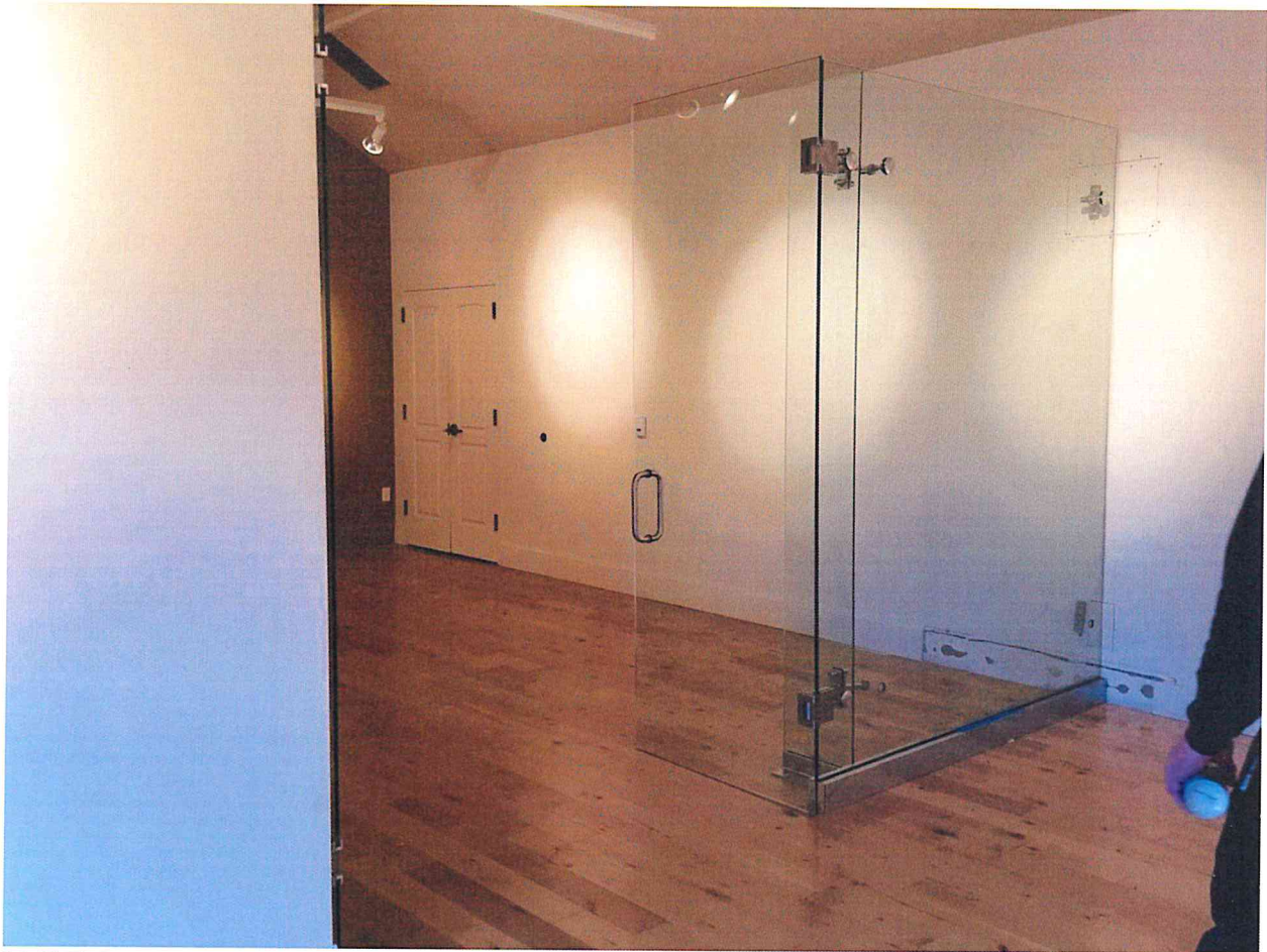
ABOVE: Demonstration glass wall system in open-door position. Hardware and installation to be similar in the proposed design.
