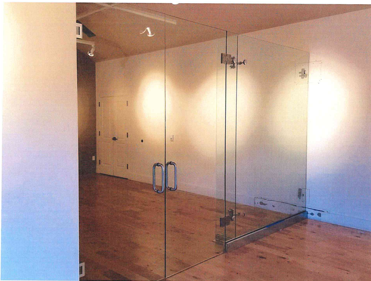
ABOVE: Demonstration glass wall system installed at Kiwi Glass office in Seaside, OR. The proposed design will be similar to this example system, but with a different base connection per next image.
